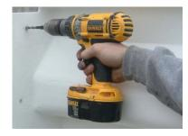
With a hammer drill and wedge drill bit, drill all pinned impression holes 2¾" deep around entire window well; sides and bottom.
