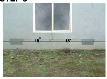
From chalk line marked in "Step 2", measure from center of window over 18" each side and attach mounting brackets with a nail gun.
