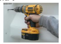
With a hammer drill and wedge drill bit, drill all pinned impression holes 23/4" deep around entire window well; sides and bottom.
