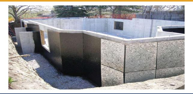
TopGun is made from a blend of 70% recycled synthetic fibers, its unique design promotes protection and effective water drainage while still retaining the boards R-value.
