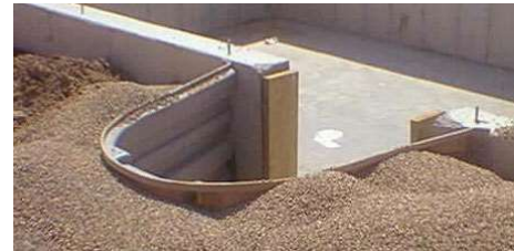
Installed Modular Well
