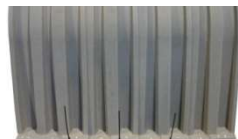
Four units wire tied.
