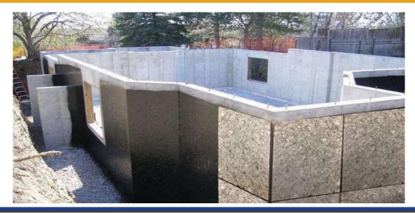
TopGun is made from a blend of 70% recycled synthetic fibers; its unique design promotes protection and effective water drainage while still retaining the boards R-Value.
