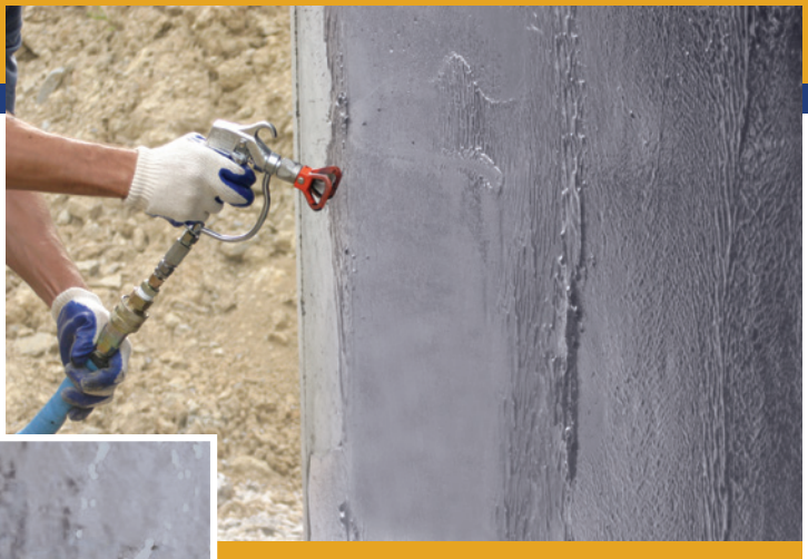
Flexible, seamless coating that seals out moisture
