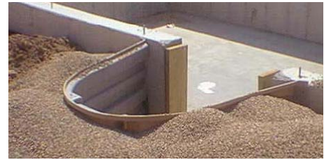
Installed Modular Well
